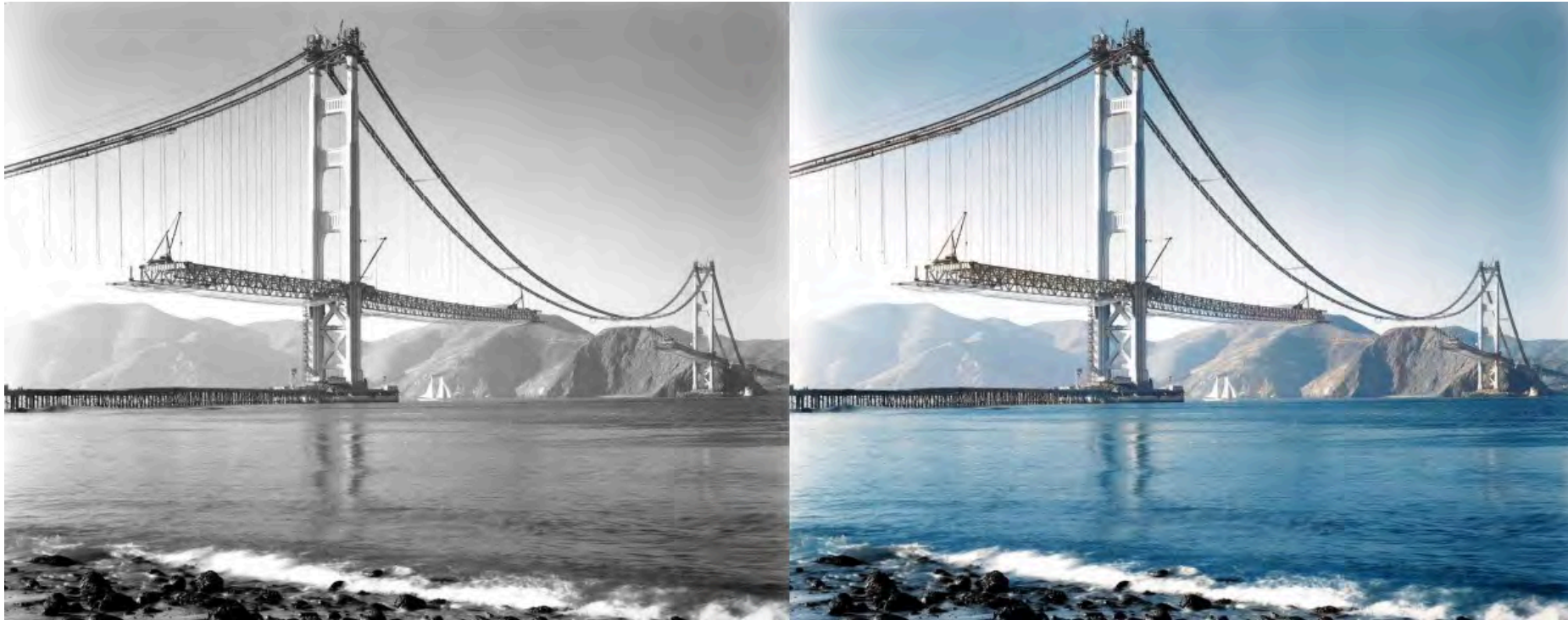
A deoldified Golden Gate Bridge under construction.
